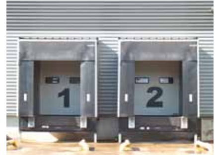
Moveable automatic truck loading docks with weather protection. Source: icmPrint.
